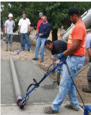
Pervious Concrete Installation Photo by: Chris Webb
