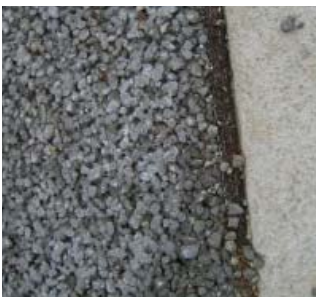
Pervious Concrete Close-up
