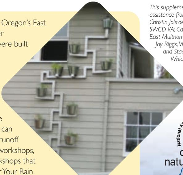
*The East Multnomah CD placed this downspout planter on their office building to absorb some of the stormwater runoff from the roof.*
