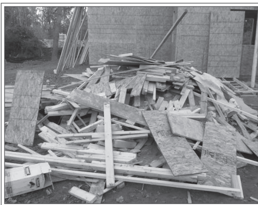
Figure 6: Unused wood from the construction of townhouses. PHOTO COURTESY OF KILEY BARNES, SOUTHERN REGIONAL EXTENSION FORESTRY.
