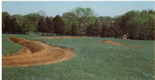
**Grassed Waterway:** This practice reduces erosion in areas where water concentrates. It should be vegetated with an adaptable grass or grass-legume mixture. Proper construction of waterways and maintenance of vegetation provide an adequate erosion free outlet in sloping fields.
