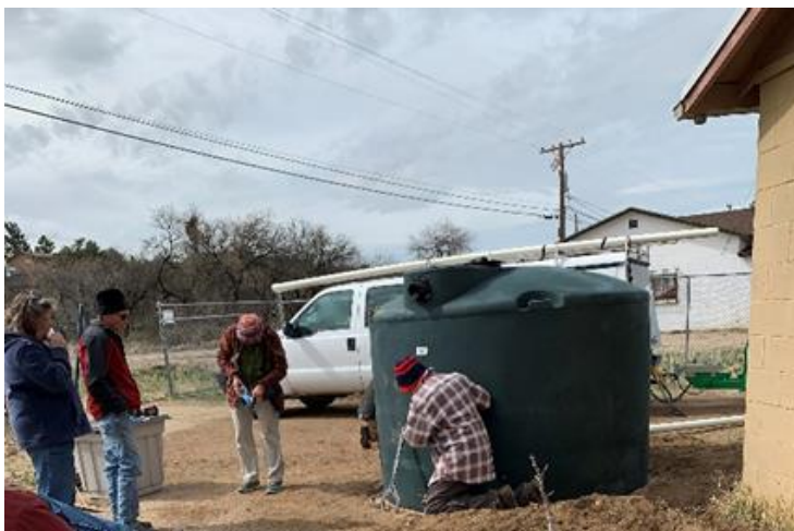
Installing the cistern
